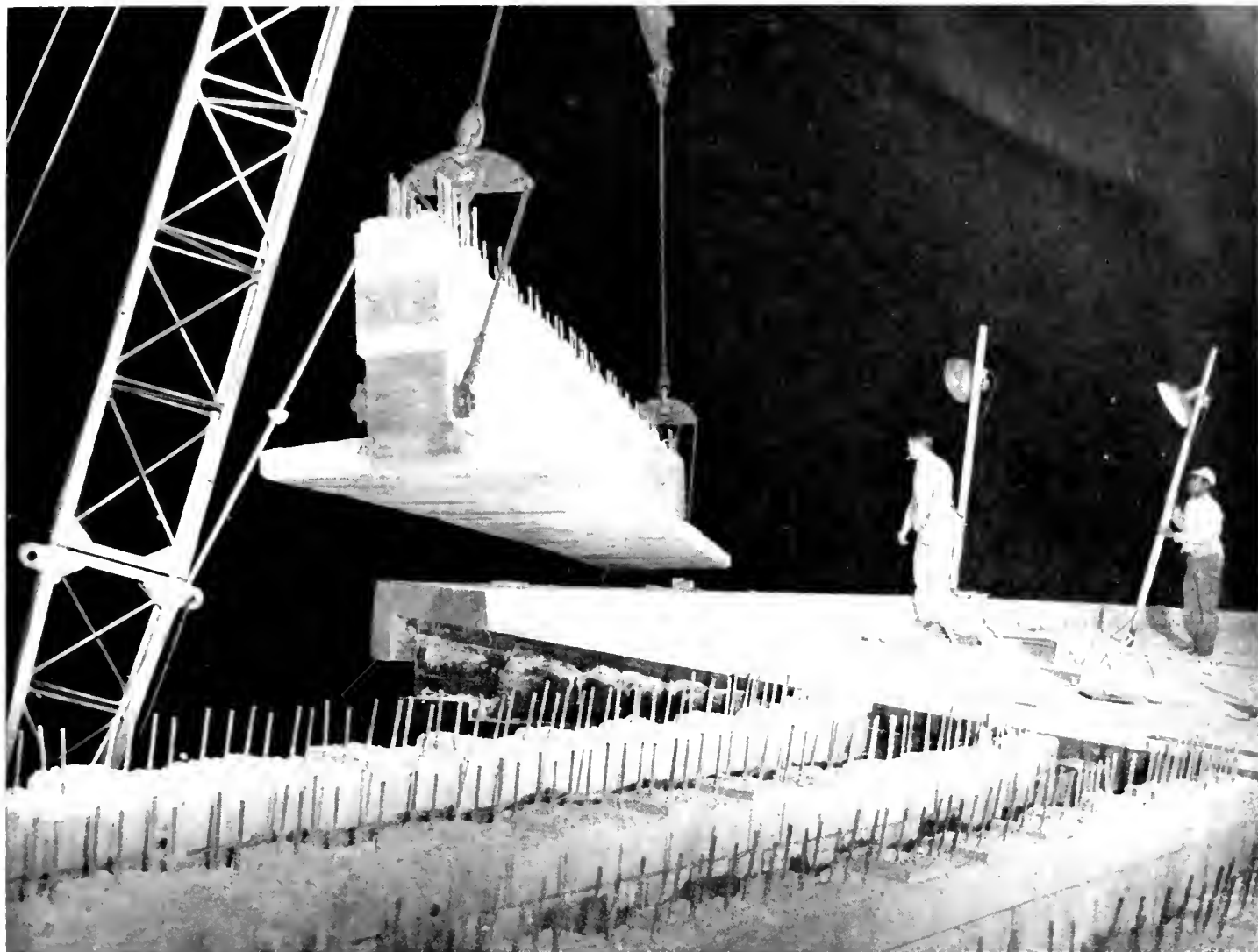
Lifting prestressed girder into place
